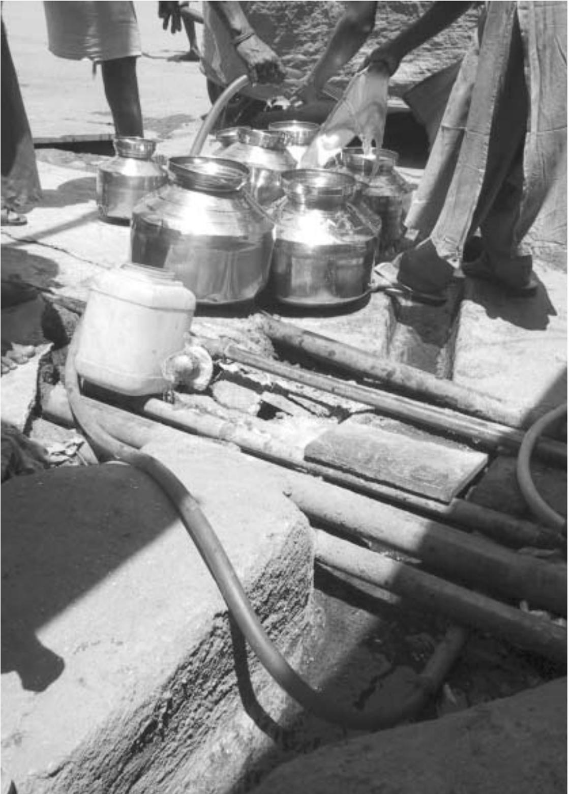
Photo 2: Tapping low-pressure piped water supplies. Credit: SPARC
