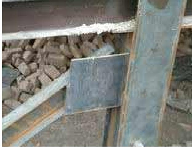
**Fig. 12: incorrectly bracing system and its gusset plate**
