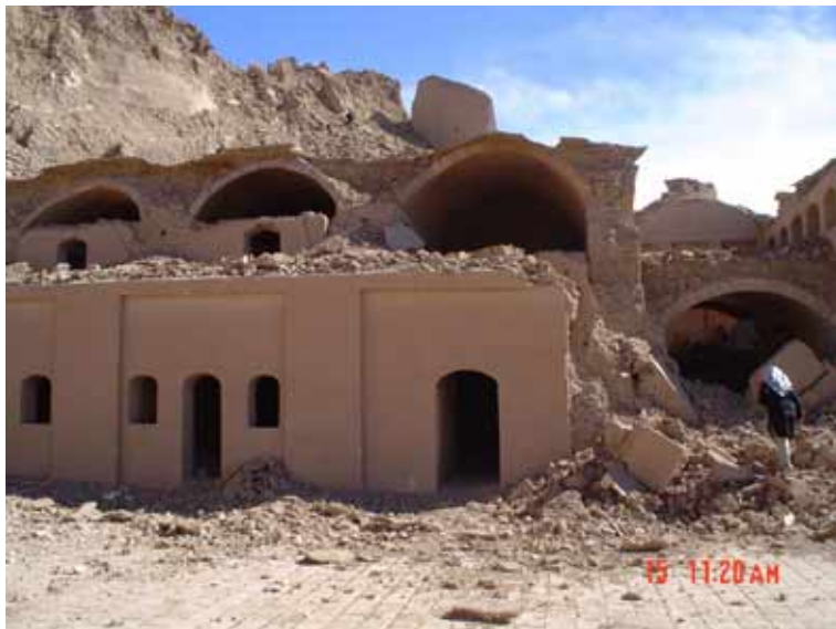
Figure 6: The north-south wall of the military barrack in Arg-e-Bam.
