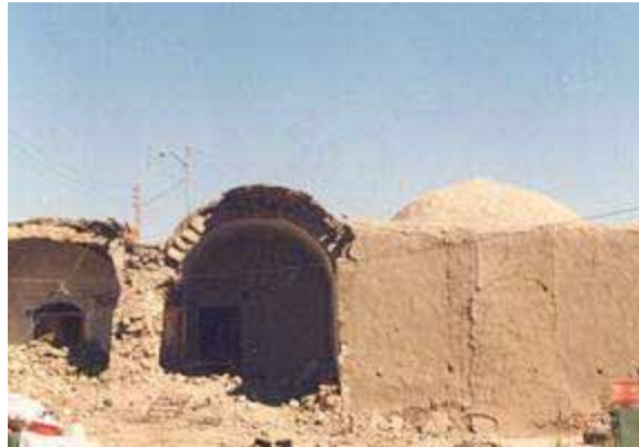
Figure 3: Typical adobe buildings with vaulted roofs in eastern Iran.
