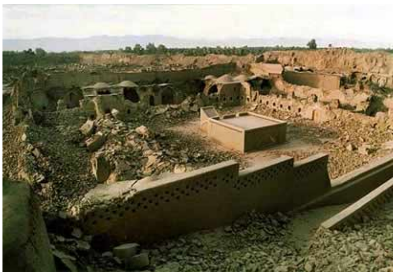
Figure 9b: A courtyard in Arg-e-Bam after earthquake.
