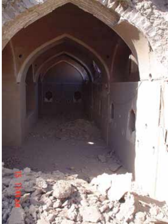
Figure 10: Vaulted roofs with arched panels
