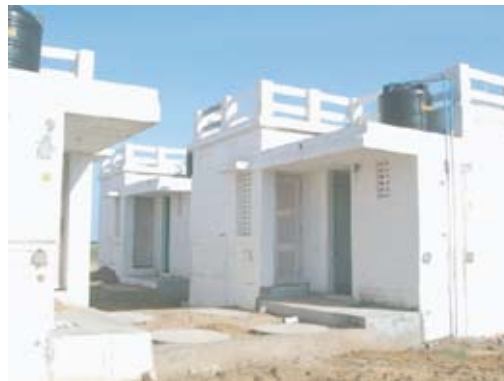
oak pit sewage system
